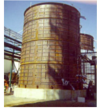
Fig. 1 Photo: ControTrace on 26' d tank at the Myerstown, PA roofing plant.
