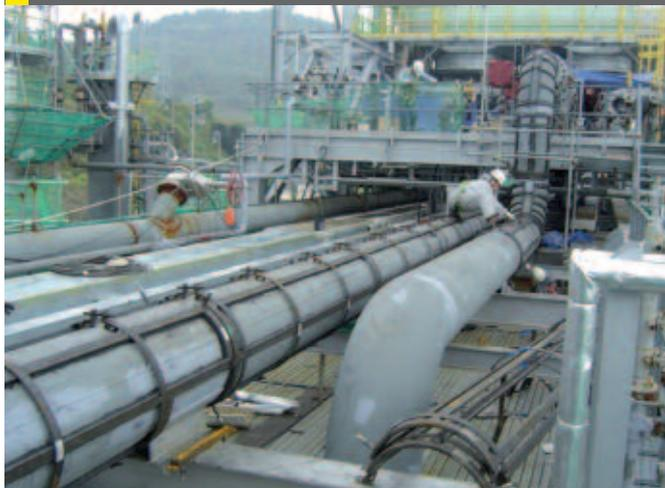
Fig 4: Tube tracing for 750 mm tail gas line
