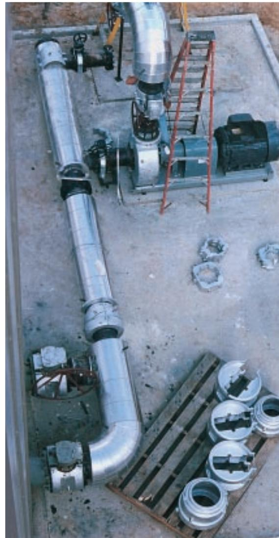
At Martin Gas' new Beaumont facility, ControHeat bolt-on jackets, like the ones pictured on the Flowserve Mark III centrifugal pump, the 12 inch Tufline butterfly and plug valves adjacent to the sulphur storage tank, and the Hyspan ball joints will be used to maintain temperature on all the process equipment. All of the 6 in., 10 in. and 12 in. transfer lines will be heated with a ControTrace thermal maintenance system.
