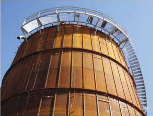
Fig 7: ControTrace panels applied to the tank roof
