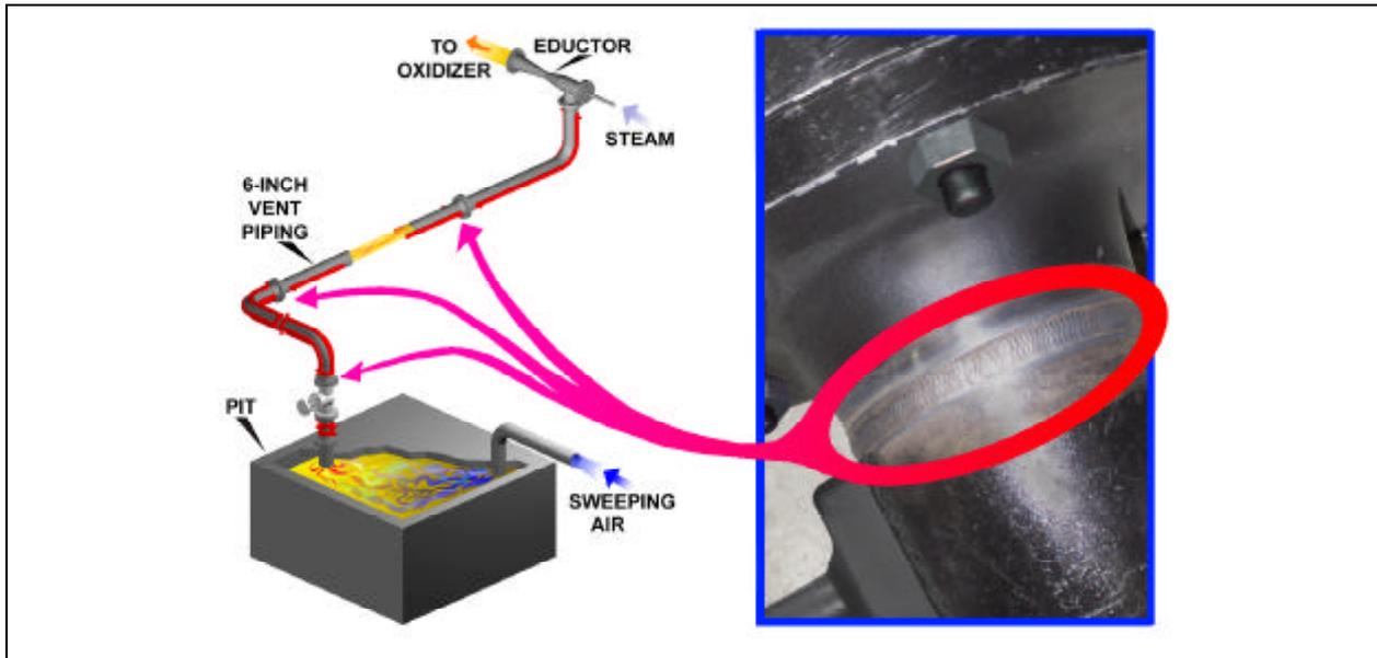
FIGURE 7 ALL PIPING WELDS CAN BE VISUALLY INSPECTED
