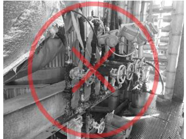
Forgotten Plant Infrastructure: The lines shown above tie into one steam trap, which results in condensate back-up and poor tracing performance.
