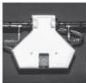
3. Bolt two halves of jacket together. Install jumper hoses.
