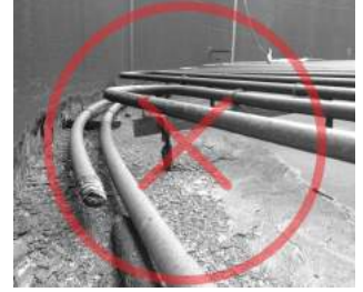
Failed Internal Coil
