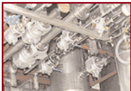
Hundreds of bolt-on jackets were used for temperature maintenance on the valves in this jacketed system.
