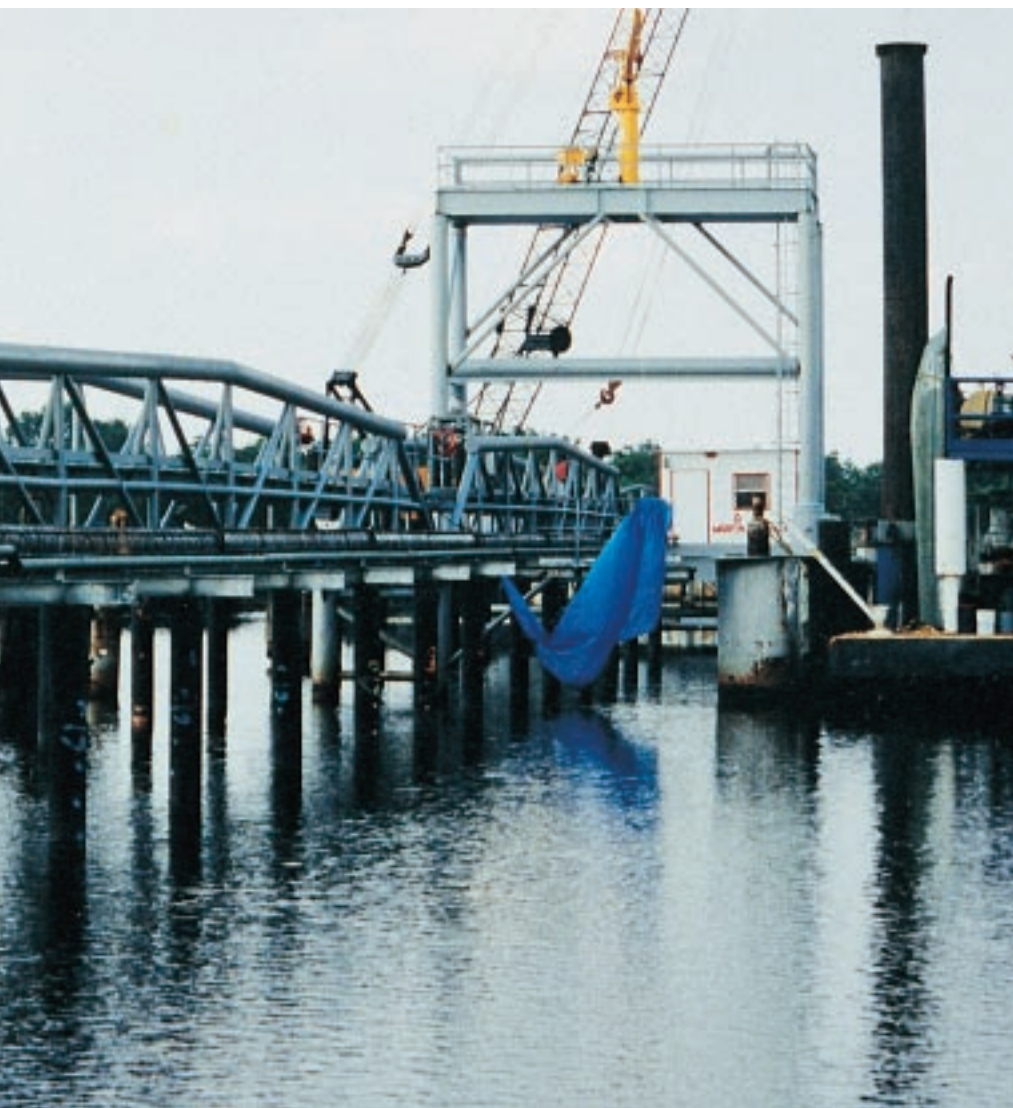
Some 1400 ft of 12 inch sulphur transfer line from the storage tanks to the barge loading area is jacketed with a ControTrace thermal maintenance system from Controls Southeast, Inc. in Charlotte, N.C.
