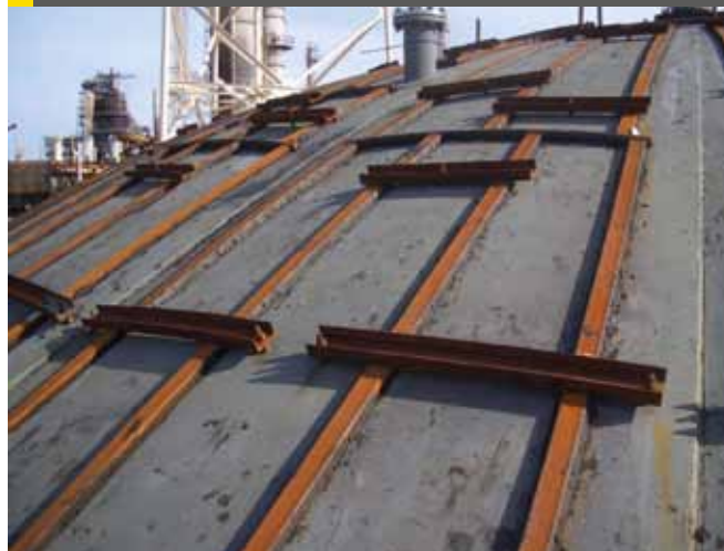
Fig 7: ControTrace panels applied to the tank roof
