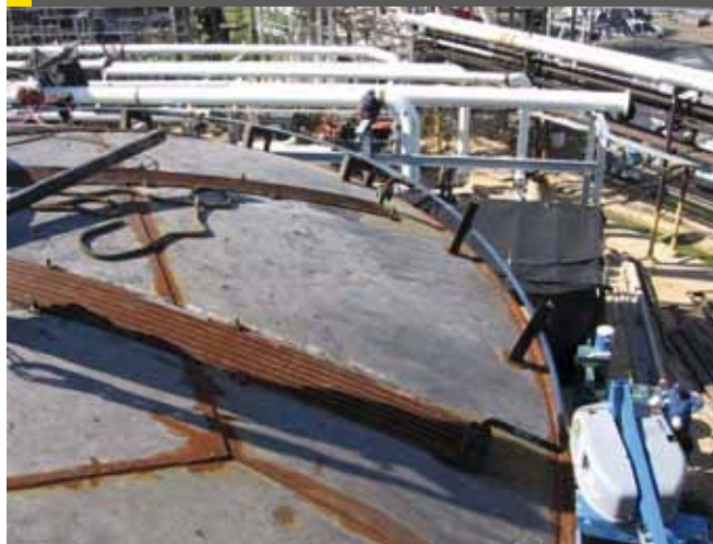
Fig 5: Exterior sheet panels applied to the tank roof
