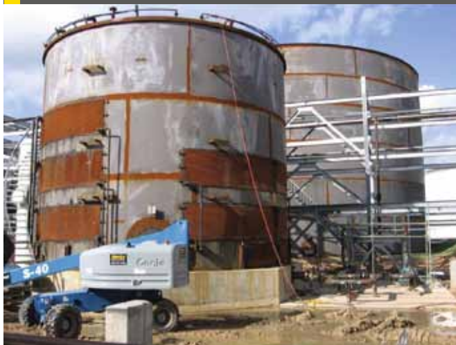
Fig 4: Exterior sheet panels applied to the tank shell
