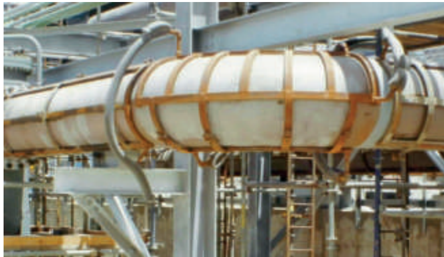
Fig. 2: Approximately four miles of Controls Southeast ControTrace® type bolt-on jacketing has been installed on this terminal’s main sulphur transfer line.
