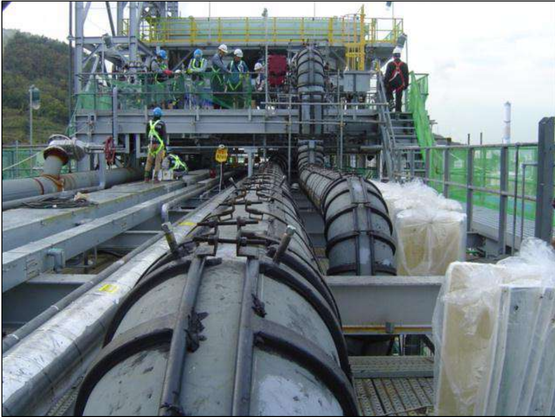
Figure 5: ControTrace Panels Installed on Large SRU Vapor Piping
